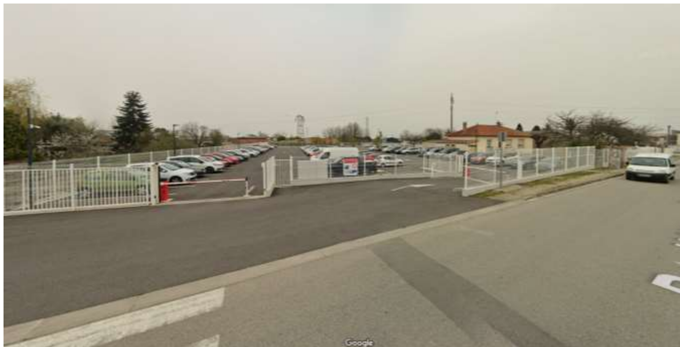
Figure 15: Photo 1 (Google Street View - Mars 2021) : Parking principal des employés
